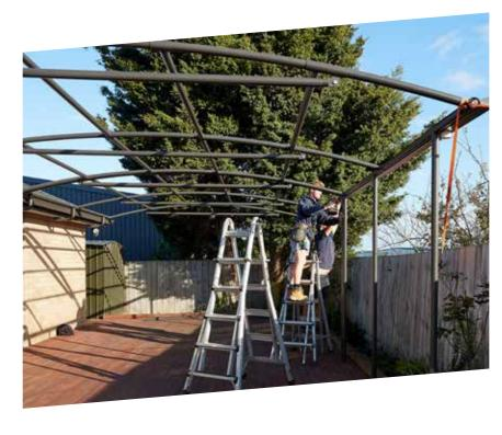
To minimise corrosion and add durability, we apply a two step powder coat system to our pre-galvanised steel. Our powder coating system resists chipping, scratching, and wear, ensuring the frame remains highly resistant to moisture/corrosion creep if damaged. We recommend regular cleaning to maintain the longevity of the frame. Hot dip galvanised finish will be supplied if the property is located in a corrosive environment or near the coast.
